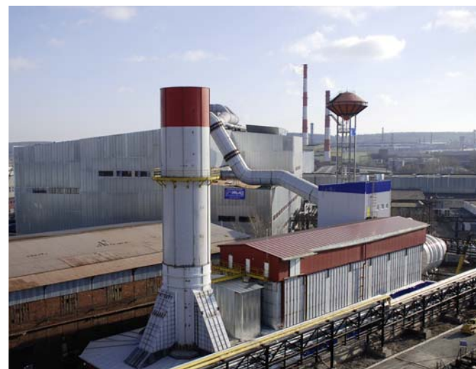
Gas cleaning system of electric arc furnace at Seversky Tube Works
