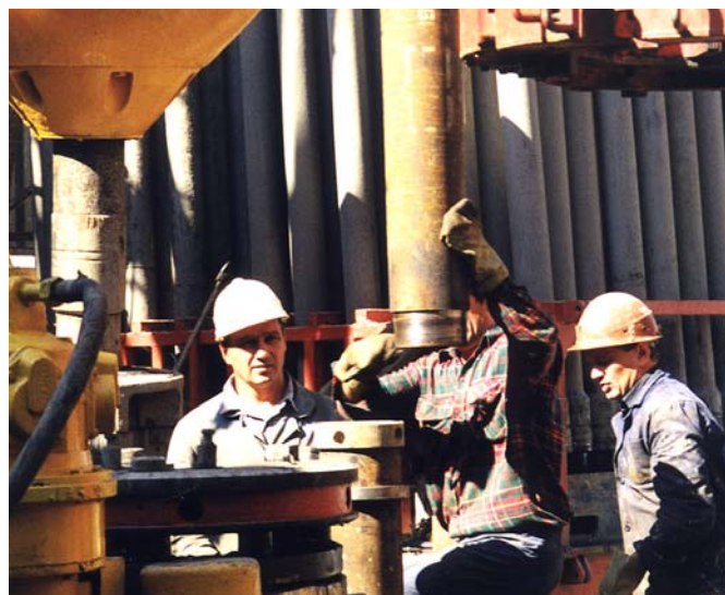
Running a drill string
