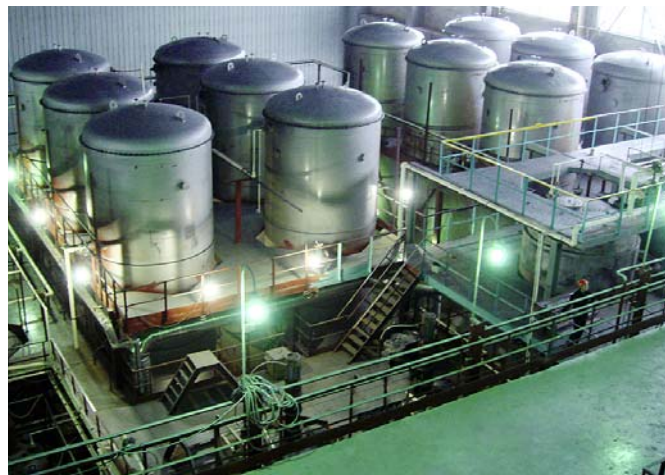
Treatment facilities at Sinarsky Pipe Plant
