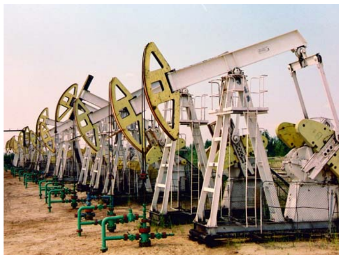
Oil pumping units
